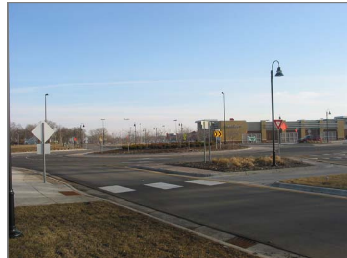
66th Street Roundabout
